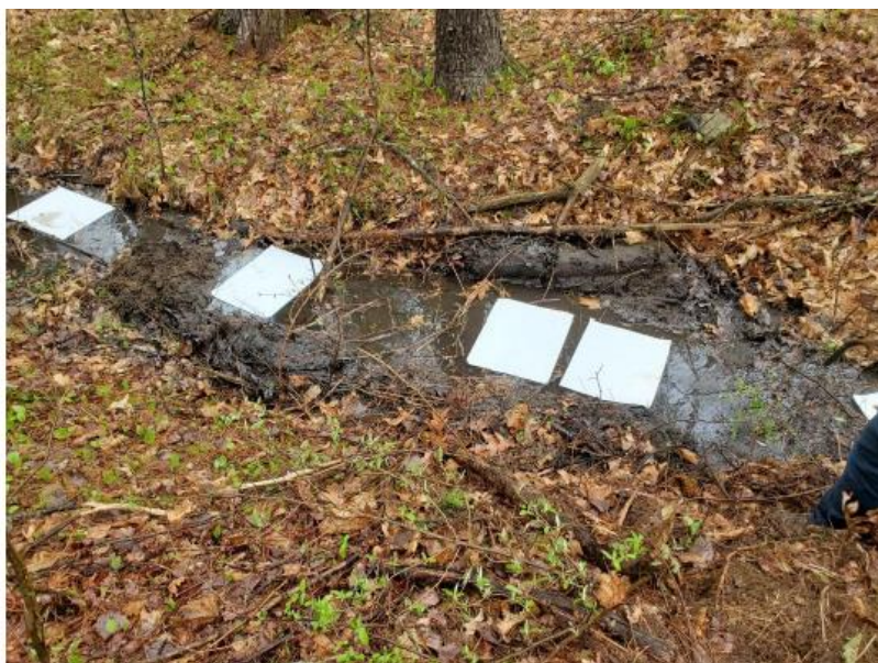
Picture 3 – Oil absorbing pads placed in flow exiting outfall (4/30/2024)
